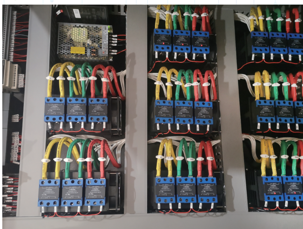
KSN series solid state relay is widely used in Mold Temperature Controller for heating control.
